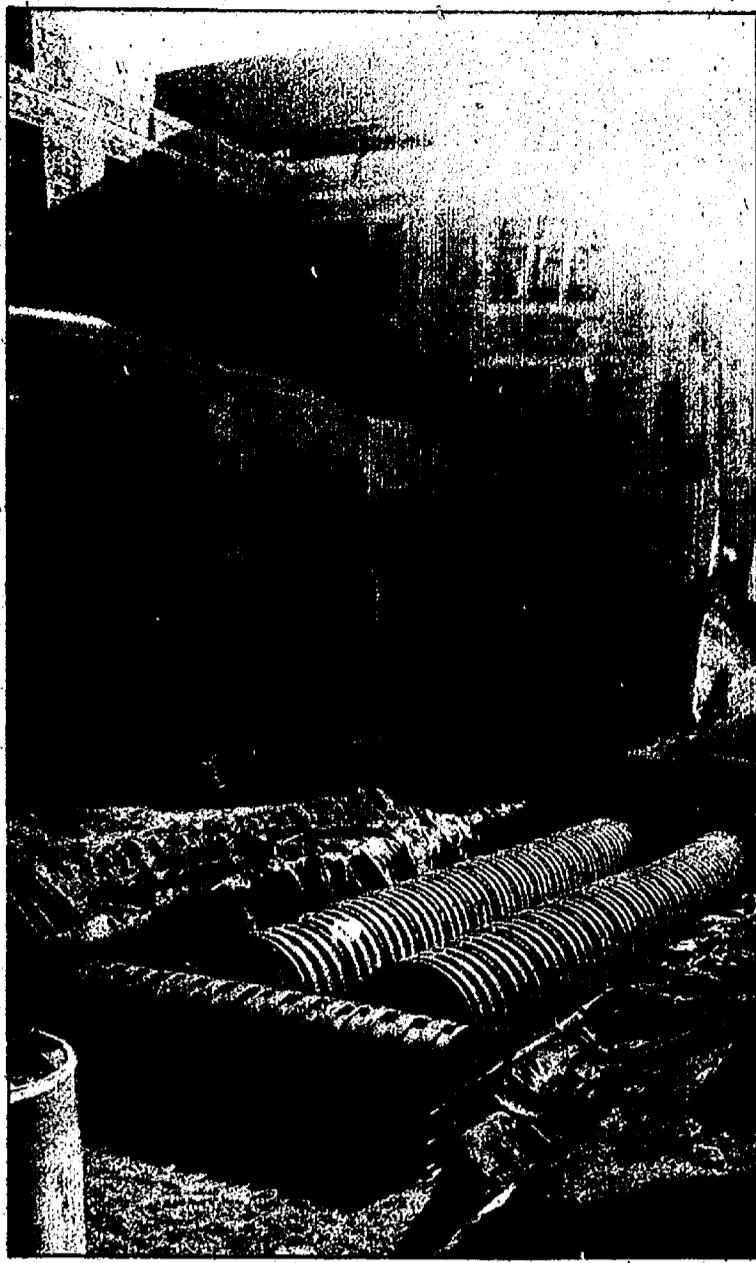
Photo courtesy of Joe Miskovich A Triton stormwater management system was installed at the University of Michigan Law School last week.
